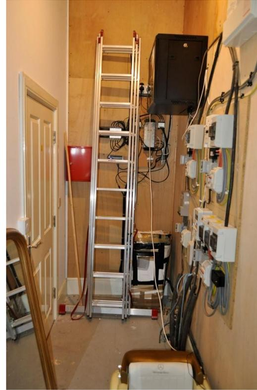
Photograph 4 – Metal ladder adjacent to electrical switch gear
