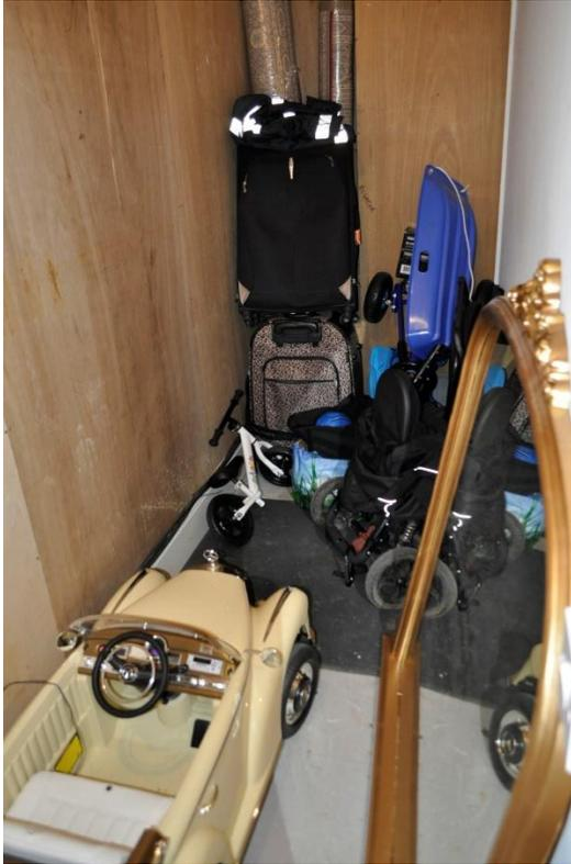
Photograph 3 – Combustible materials in electric intake room
